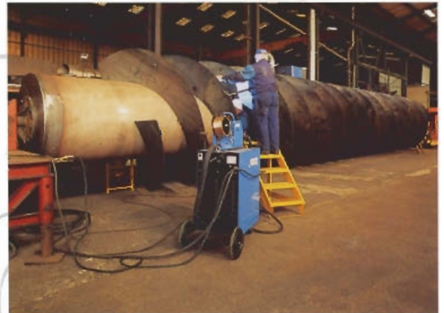
Soudage des spires Welding the flights
